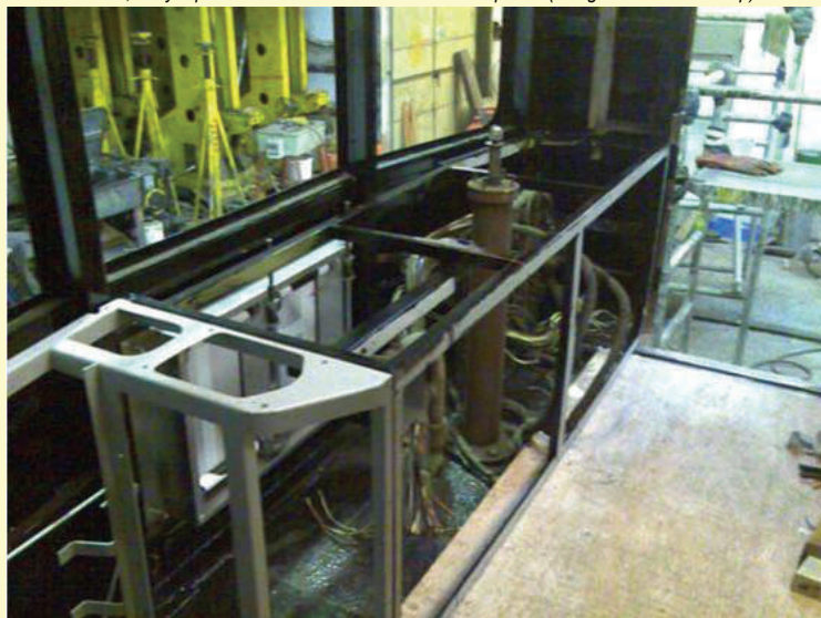
56097, the refurbished cab desk frame now fitted (Llangollen Railcar Group)
